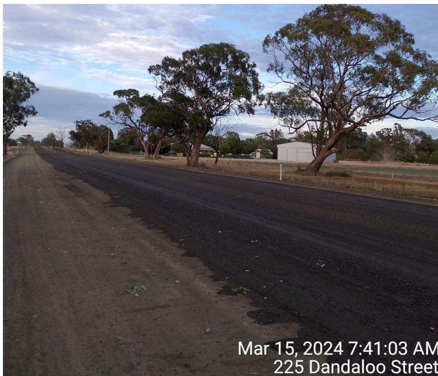
Figure 4: Dandaloo Street has been ressealed
