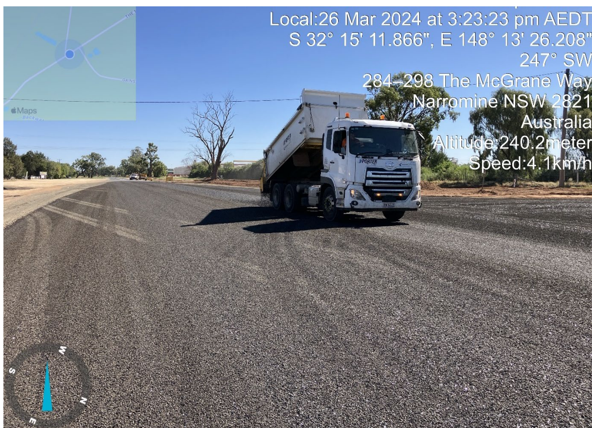
Figure 3: Sealing of McGrane Way / Gainsborough Road Intersection
