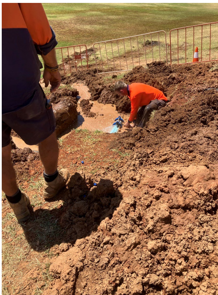
Figure 2: Parks and gardens staff repairing an irrigation main pipe leak
